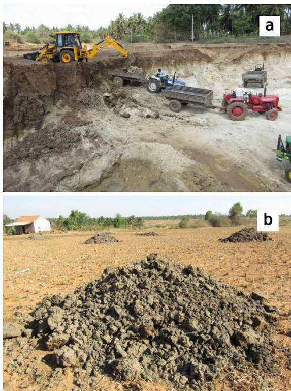
Figure 1. (a) Desilting of water harvesting tanks using machine (b) Tank silt
