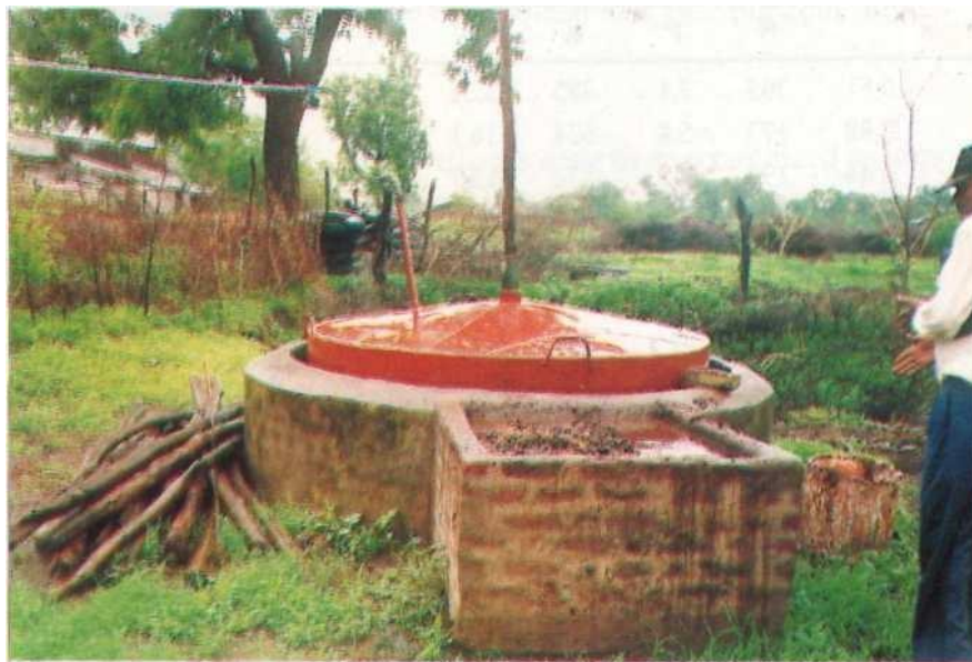
Plate 3 : Gobar gas plant in operation at farmers home
